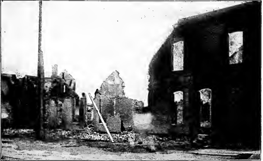
VIEW IN THE CITY OF MEXICO, MARCH, 1913.
